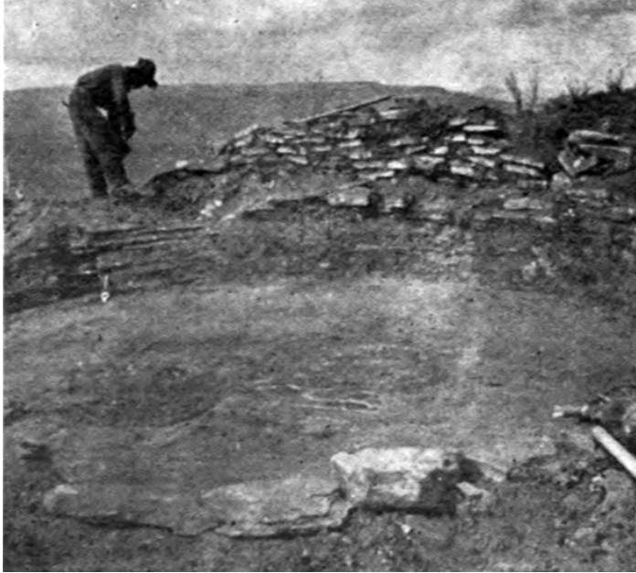
FIGURE 12b. The Guard House during excavations by Jeançon (Jeançon 1922).
