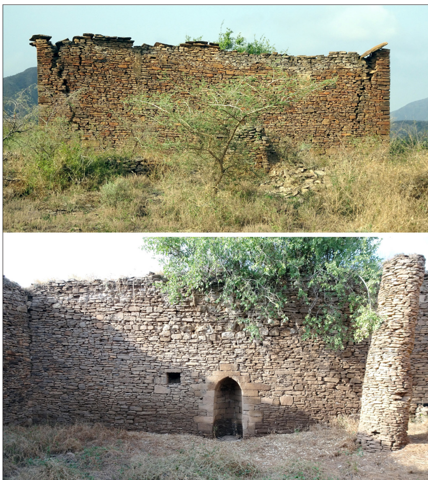
Figure 14. Top. Exterior of the mosque at Nora. Bottom. Interior of the mosque at Nora showing the mihrab and one of the columns that would have supported the roof (photos. T. Insoll).
