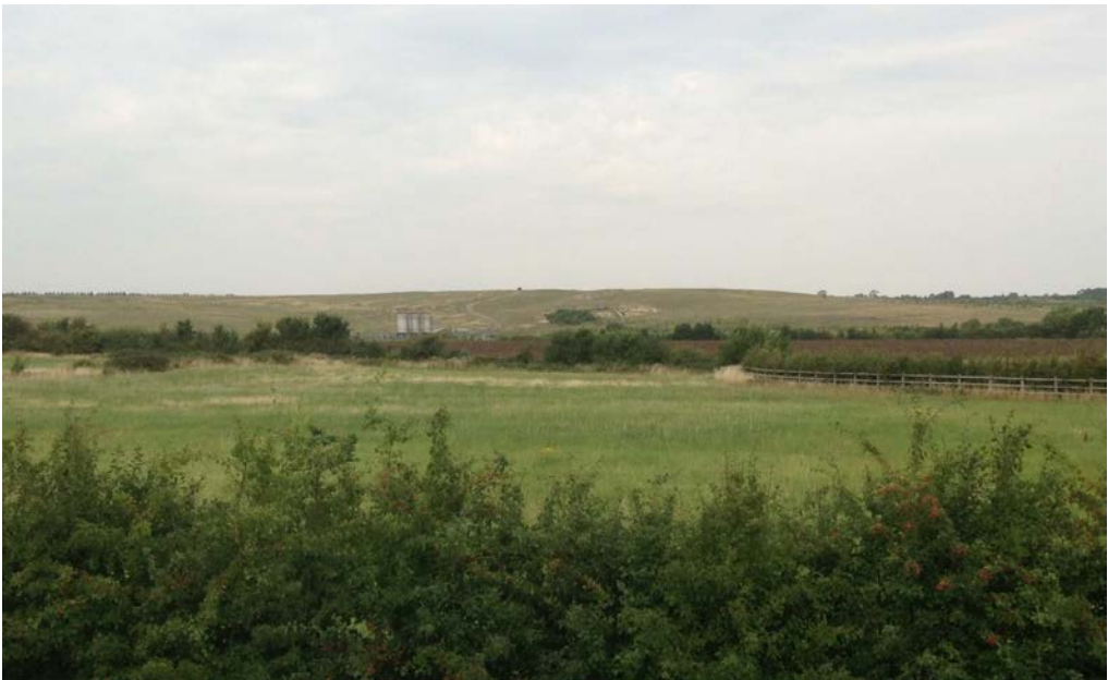
FIGURE 1. Landfill hill at Brogborough, viewed from the A421 looking west. A small methane-processing plant is visible. Everything above the general lie of the land is sculpted from landfill. Below the highest point on the hill is about 50 m of compacted waste material.
