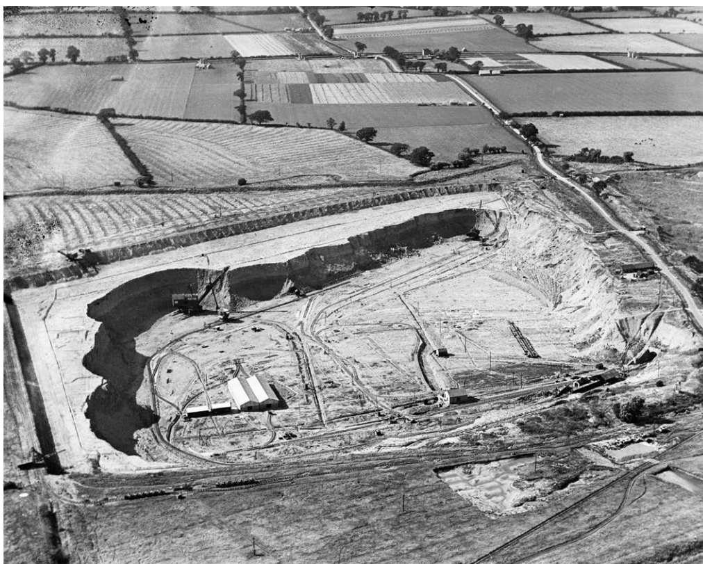
FIGURE 3. Extraction of clay by drag-line excavator, 1930s–1940s, pit near Stewartby, Bedfordshire (Britain from Above, © Historic England).
