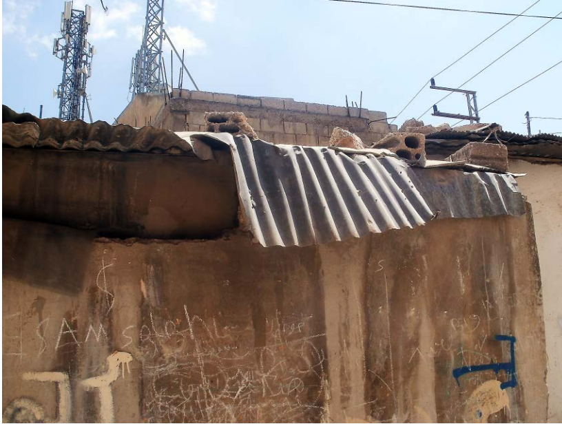
FIGURE 3. Zinc roof, Talbīyah Camp (photograph by authors).
